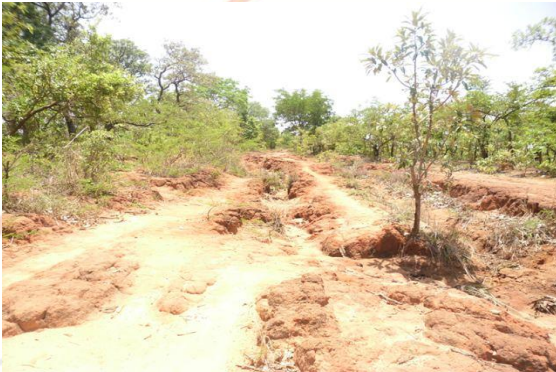
Tungan Jika Road before intervention
